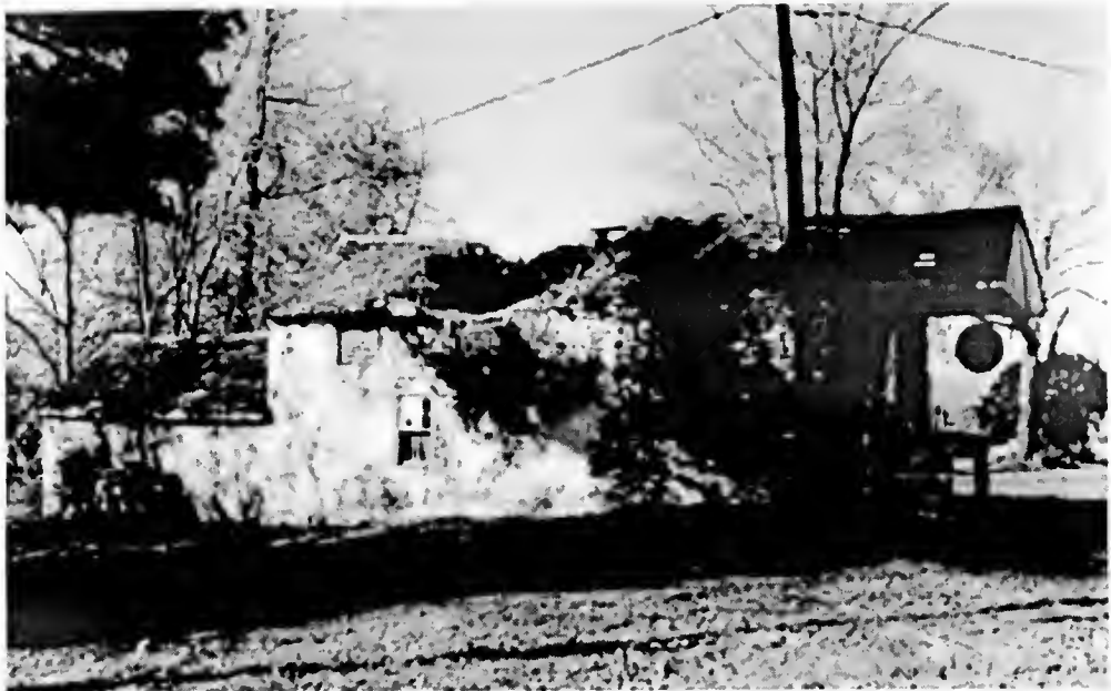
Figure 44 Smokehouse/Root Cellar, looking north, 2001
